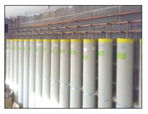
The Be-Green energy storage cells store heat in a petroleum gel, a method so efficient that it only loses one degree of heat every 18 hours. The system has a life expectancy of over 100 years and does not require any mechanics or electrics, the cells only have flow and return pipes and can be installed and hidden anywhere in the house, garage, ceiling or floor.
